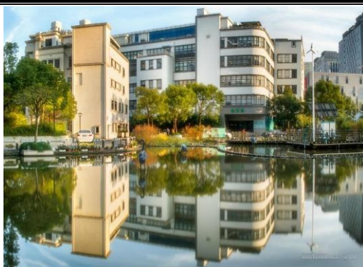
The former Union Brewery has become Mengqing Garden.
